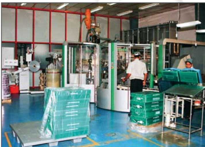
Laminate Tube Making Facility
