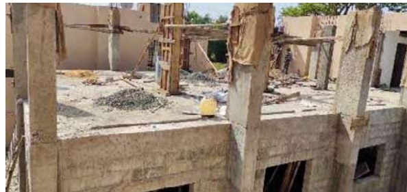
Construction of new classrooms at Dhanoli Primary School, Vapi
