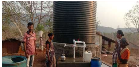
Drinking water facility for villagers in Madh & Sarmal villages
