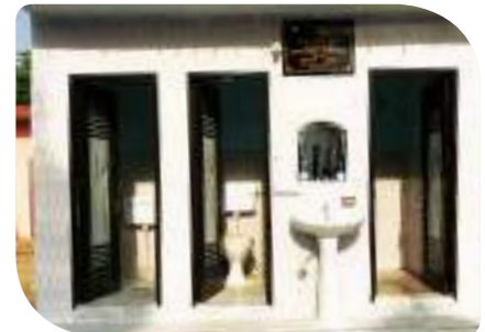
Public Lavatory in Nalagarh, Himachal Pradesh
